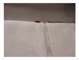
Screw board in place while mud is still wet. If edges pop up between screws staple like vinyl corners.
