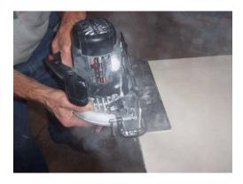
Run saw along butt edge face side.
