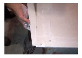
Butter EZ Taper wedge with mud and insert into slot, thick edge first
